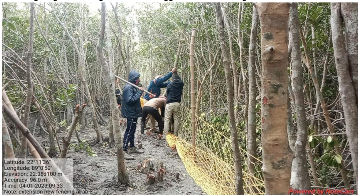
Figure 22. Nylon net fencing in Sundarban (Source: Sundarban Tiger Reserve).
